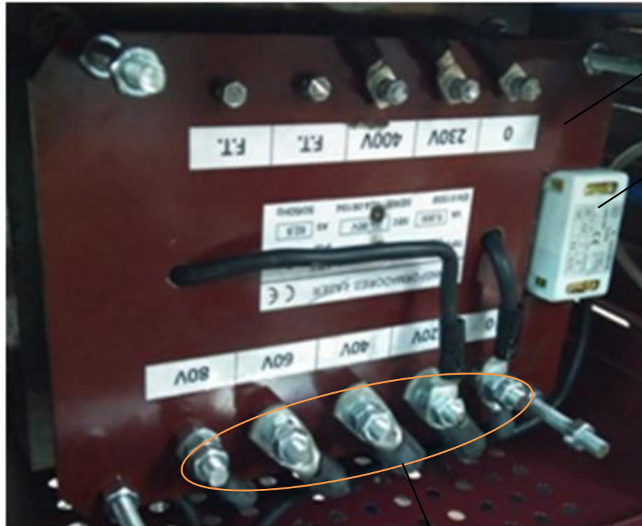
5000 VA transformer connection example
